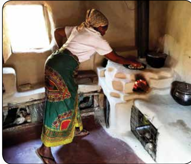
The Nandi women designed a cook stove so that it is elevated, so the woman doesn’t have to bend over the stove to cook. They also built a coop under the stove to act as an incubator to raise chicks to be able to sell chickens at the market.
