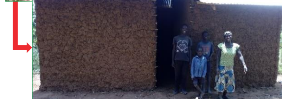
A widowed caregiver of 3 OVC from Busia County renovated her collapsed home with USAID 4TheChild Emergency Support Fund.
